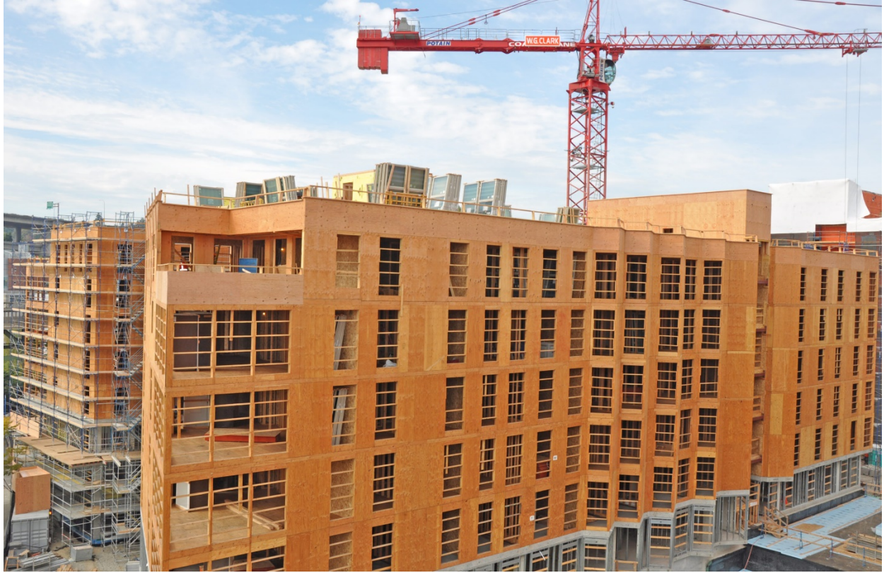
Figure 4: Podium Construction. This image is an example of a podium construction building under construction. The first story is concrete and the five stories above are wood frame; typically, light weight wood I-beams are used as the floor and roof supports.
